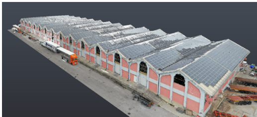
Survey of exterior parts of the Warehouse nr.71 (point cloud)
